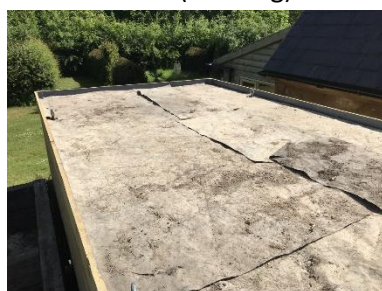
Filter layer of geotextile
