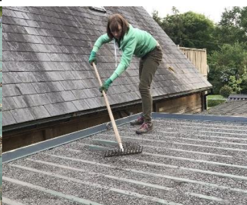
Adding drainage/water layer
