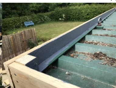
Enclosing the roof
